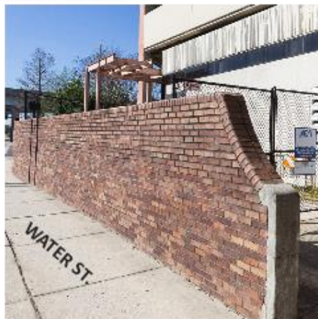
Security fencing and pumping station brick wall
